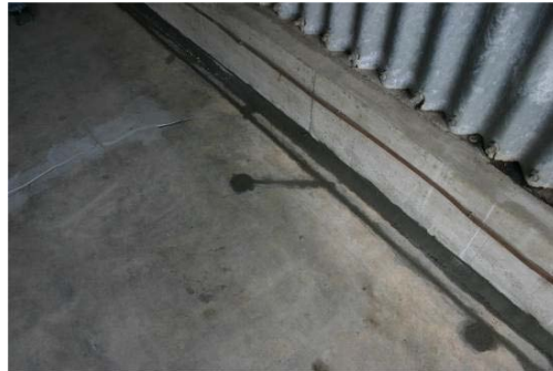
Completed grouting of cables
