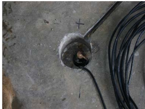
Installation of cathode rod
