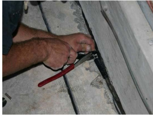
Anode installation
