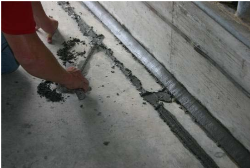
Grouting embedded cables
