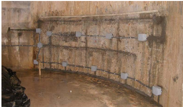
Figure 42. Completed installation with junction boxes and conduit.
