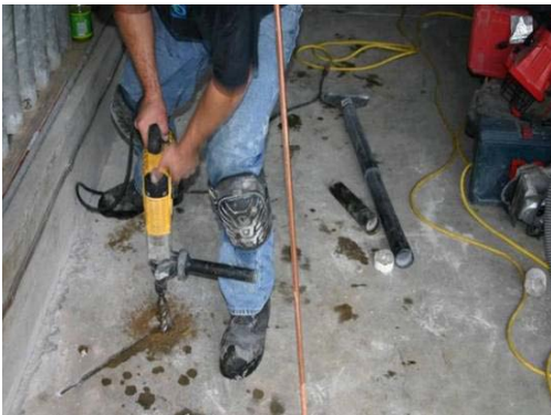
Drilling hole for cathode
