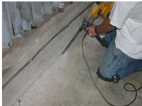
Chipping out groove for anode installation
