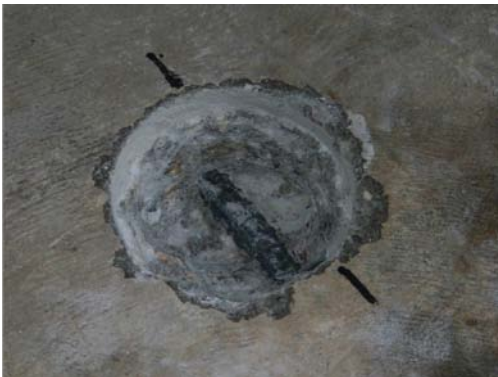
Exposed rebar
