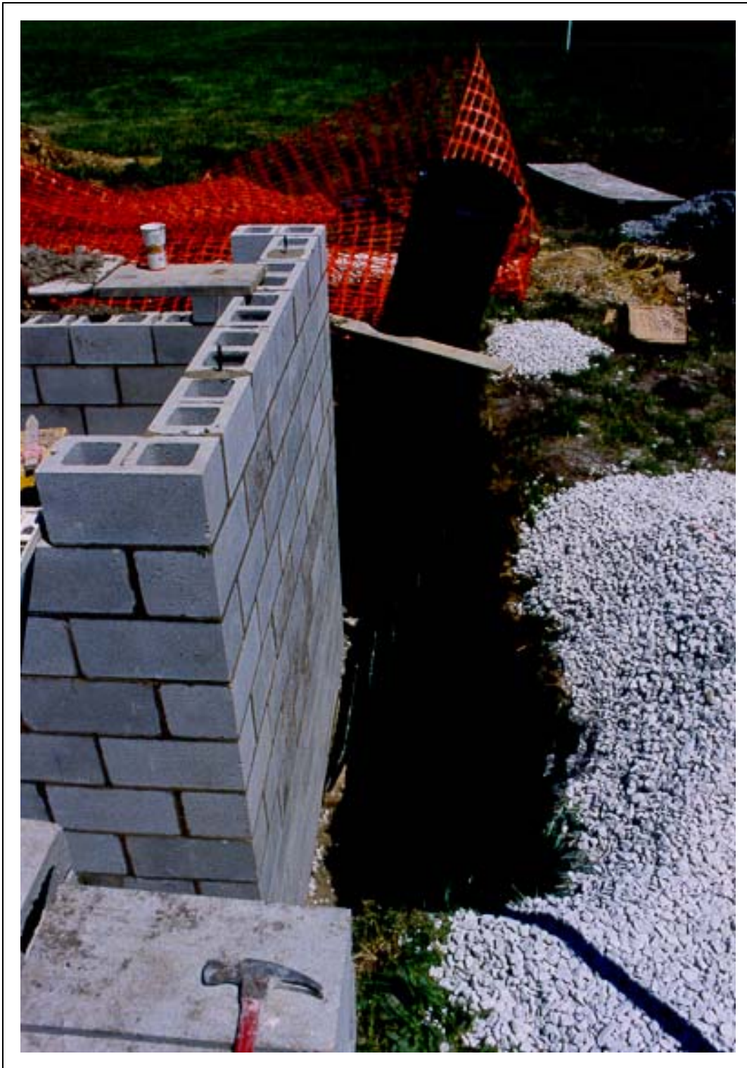
Figure D8. Detail of trench surrounding the block basement including 24-in. (60.96 cm) drain tile.
