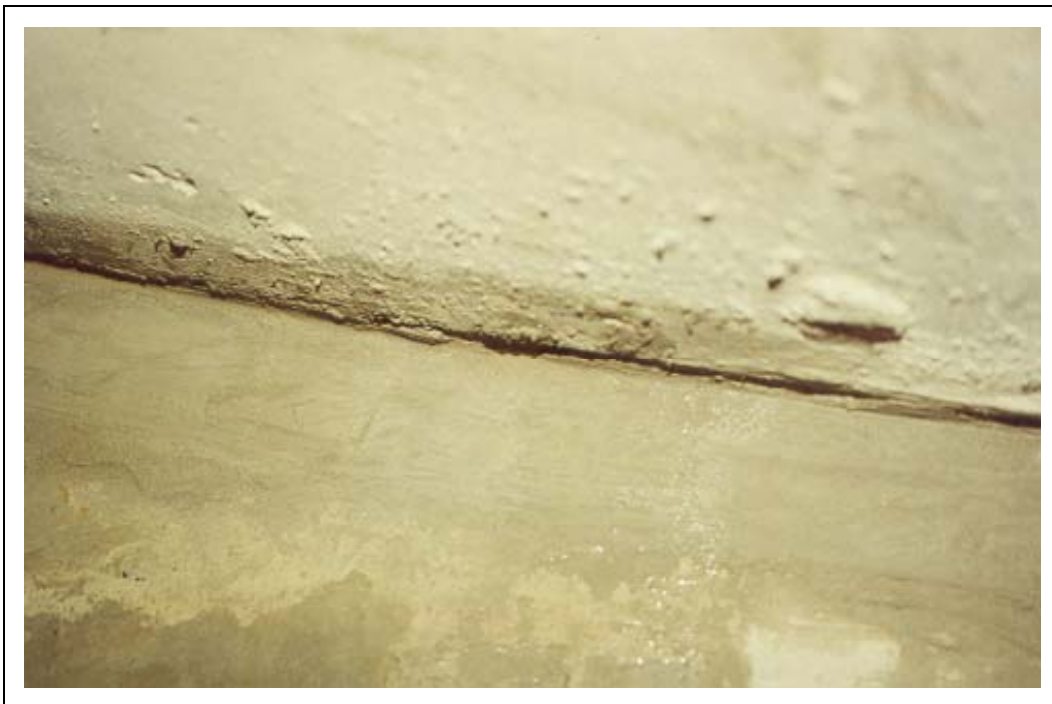
Figure D24. Finished wall-to-floor joint, ready to cure in the concrete basement.
