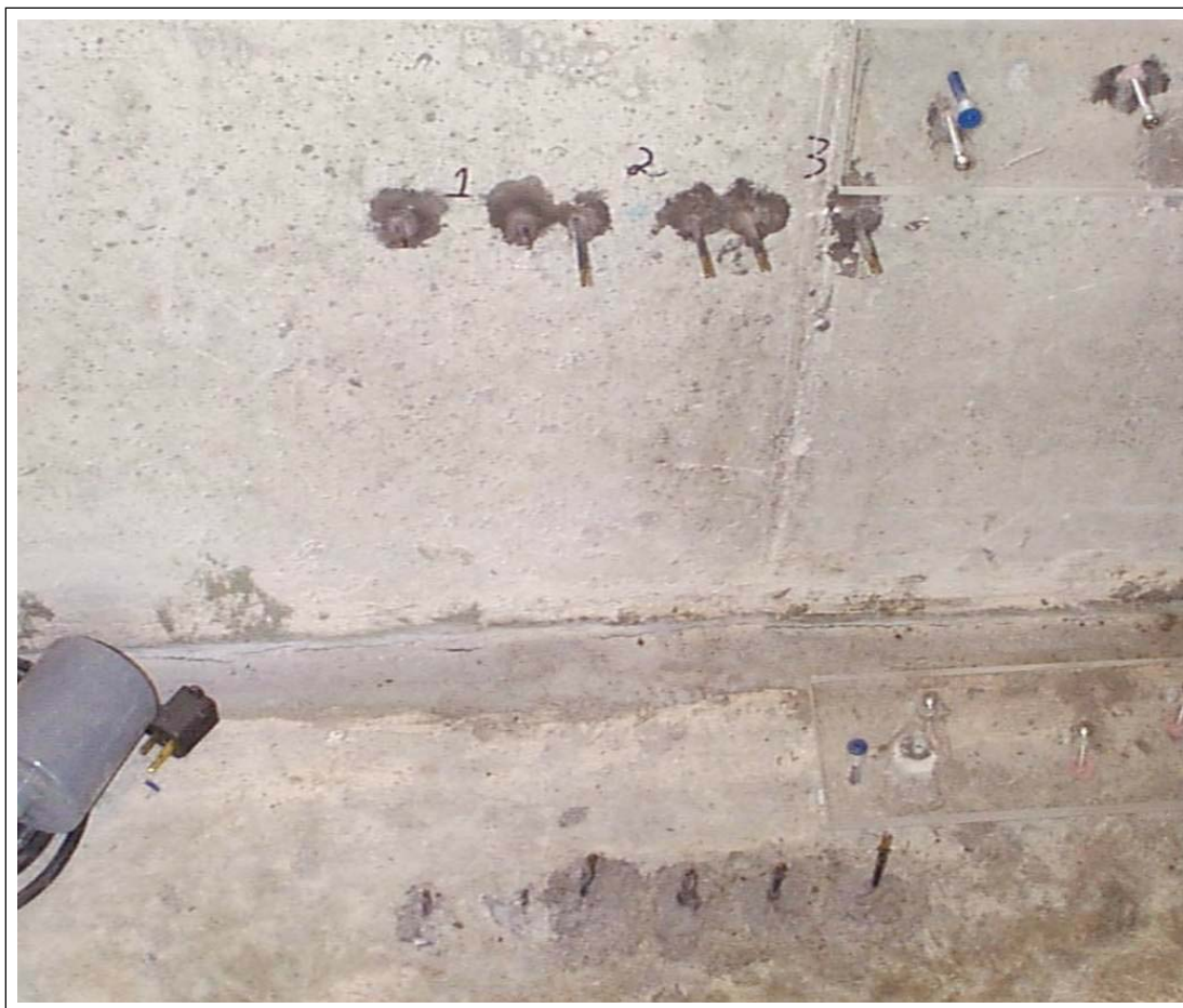
Figure 59. Typical cold joint condition in concrete basement after EOP system was operating.
