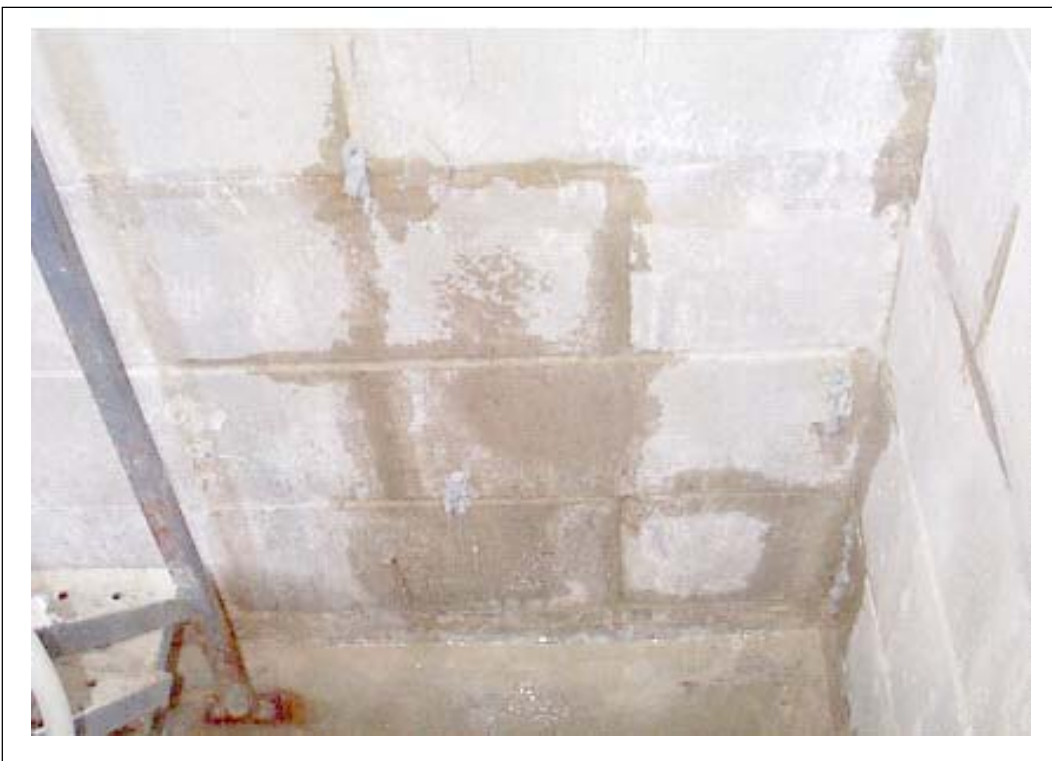
Figure 66. Collected water at the bottom of the block basement; note the seepage through the block face as well as at the joints between each block.
