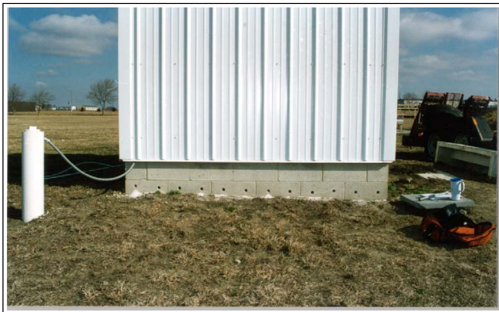
Figure 51. South wall of block basement above grade showing holes for filling wall with grout.
