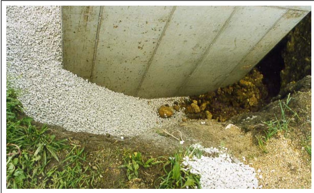
Figure D6. South wall of concrete basement. Clear view of gravel backfill extending from the West wall to the south wall. A small amount of the clay backfill is visible from the eastern wall.
