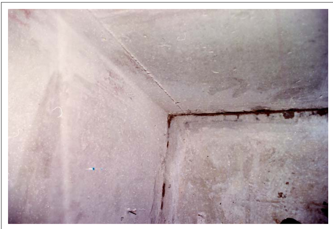
Figure 58. Close-up of weeping cold joint in concrete basement after repair dehumidification.
