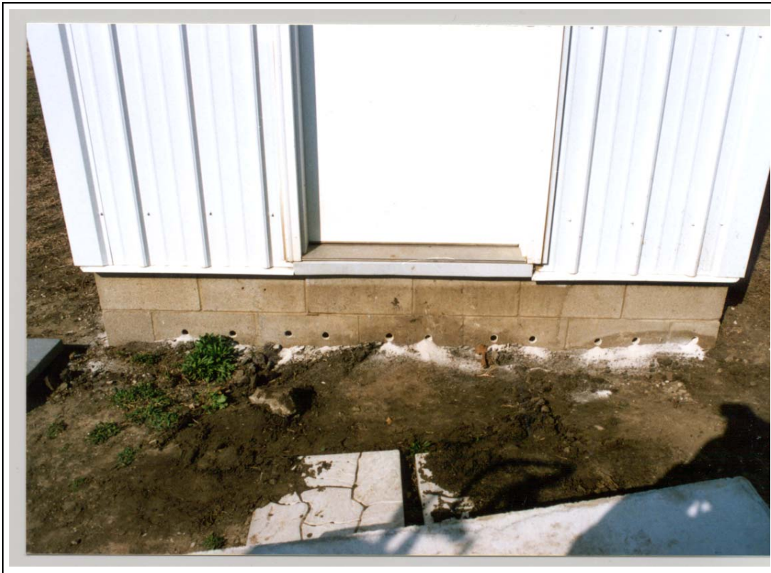
Figure 52. East wall of block basement with above-grade holes drilled to fill wall with grout.
