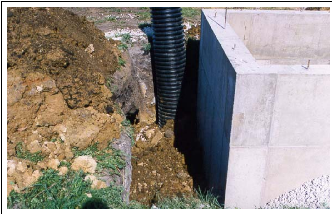
Figure D4. Note the 24-in. (60.96 cm) drain tile used to deliver extra water to the concrete basement footer. Similar drain tile was installed in the block basement as well.
