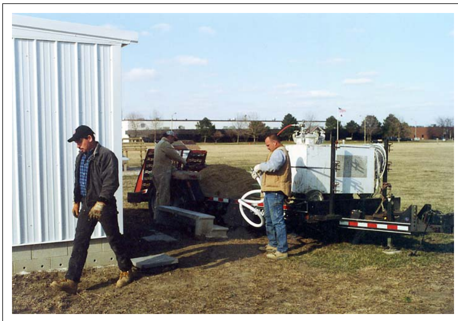
Figure 64. Overview of grout pumping machinery.
