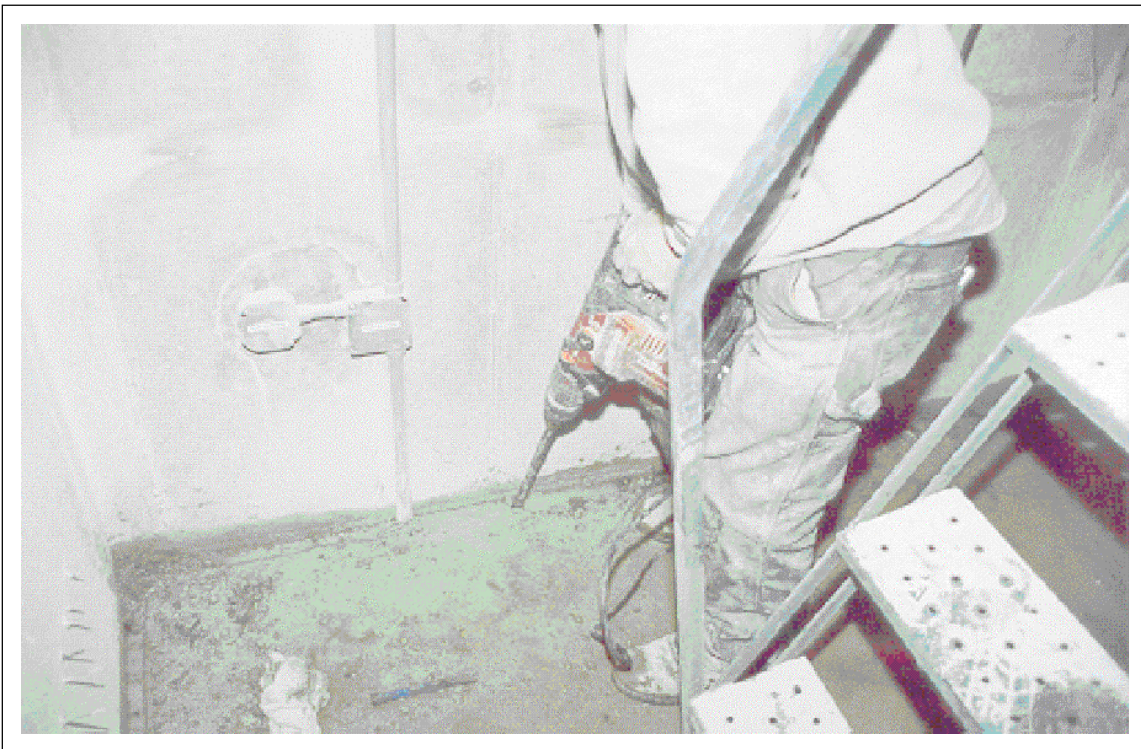
Figure D22. Electric powered chisel used in concrete basement to finish the cut area at the joint prior to application of hydraulic cement.
