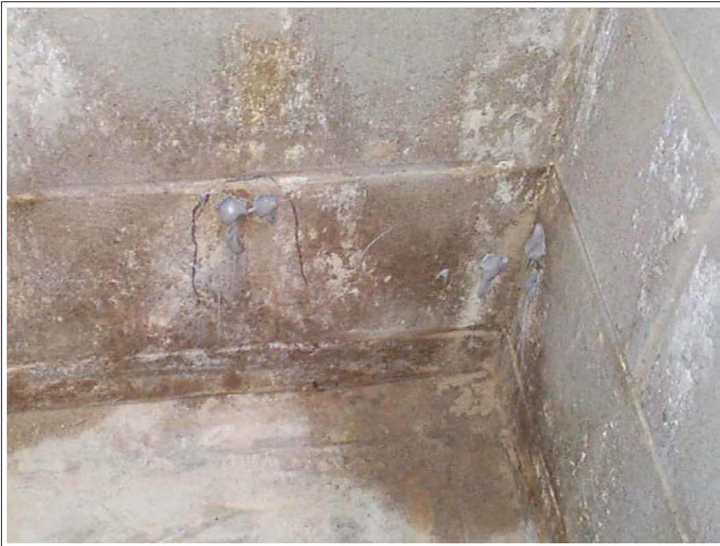
Figure 65. Close-up of wall-floor joint in block basement after epoxy injection.
