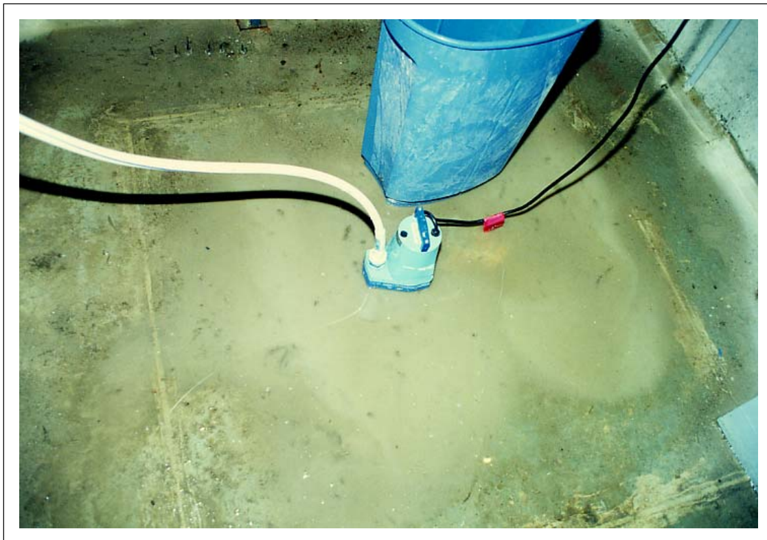
Figure 55. Active water from the cold joint is being pumped down (concrete basement as built).
