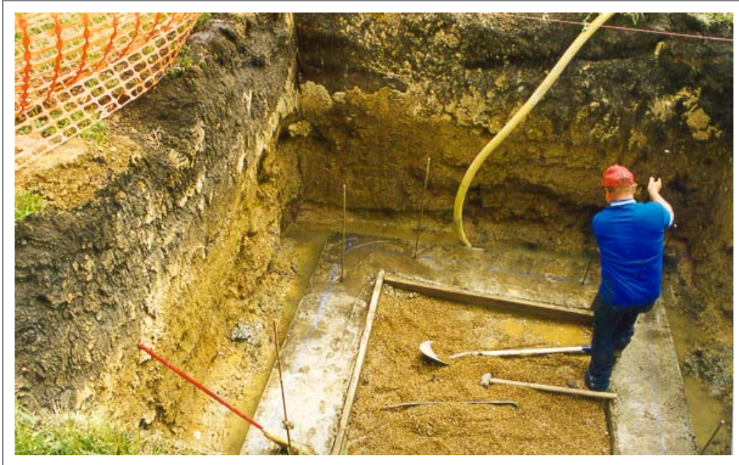
Figure D1. Footer of concrete basement cured, work in progress to set the wall forms.
