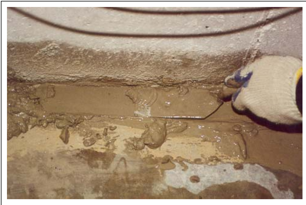
Figure D23. Hand application of Waterstop, a hydraulic cement, in concrete basement.
