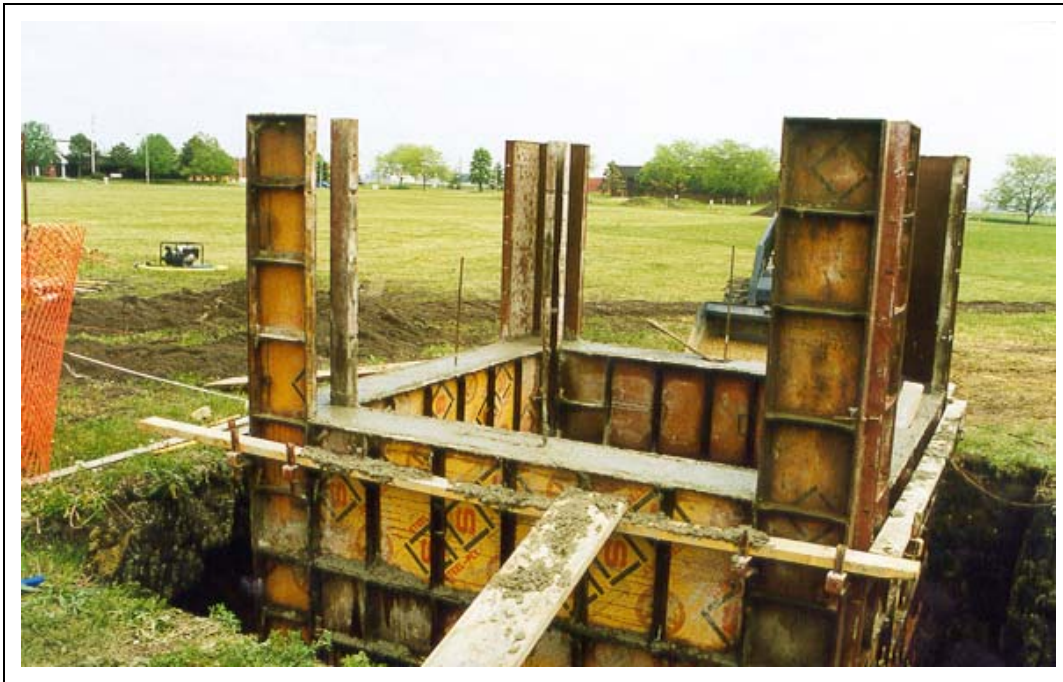
Figure D2. Concrete basement wall forms erected.
