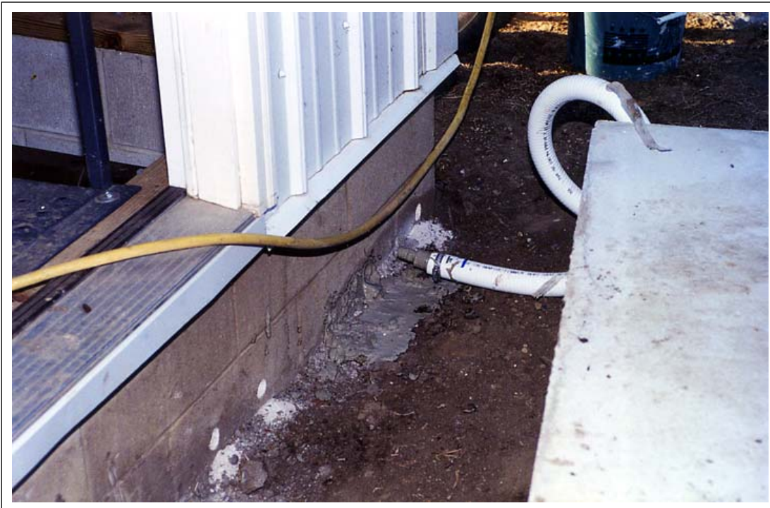
Figure 63. Showing grout pumping in progress on the Block Basement.
